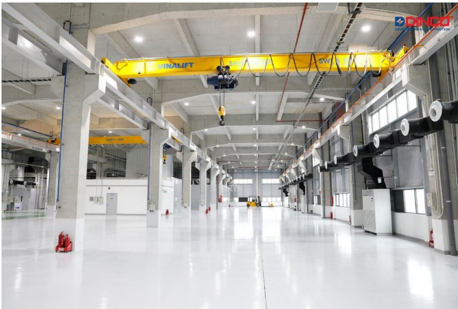
Figure 5. A manufacturing plant in Vietnam was built with a robust structural system, including beams, columns, and floors. Source: DINCO E&G
